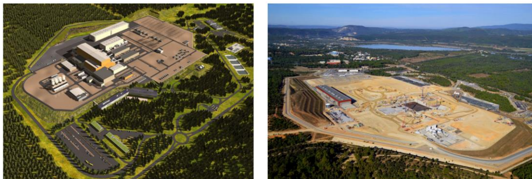
Figure 2.16 The site where ITER was built (a) the form of architectural design and (b) the original construction (Dubus, 2014)
